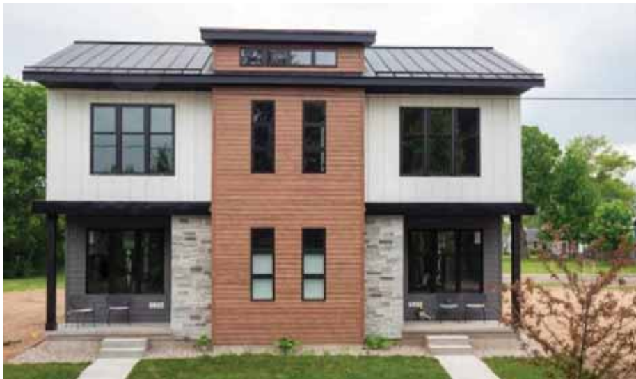
Recently constructed twin home
