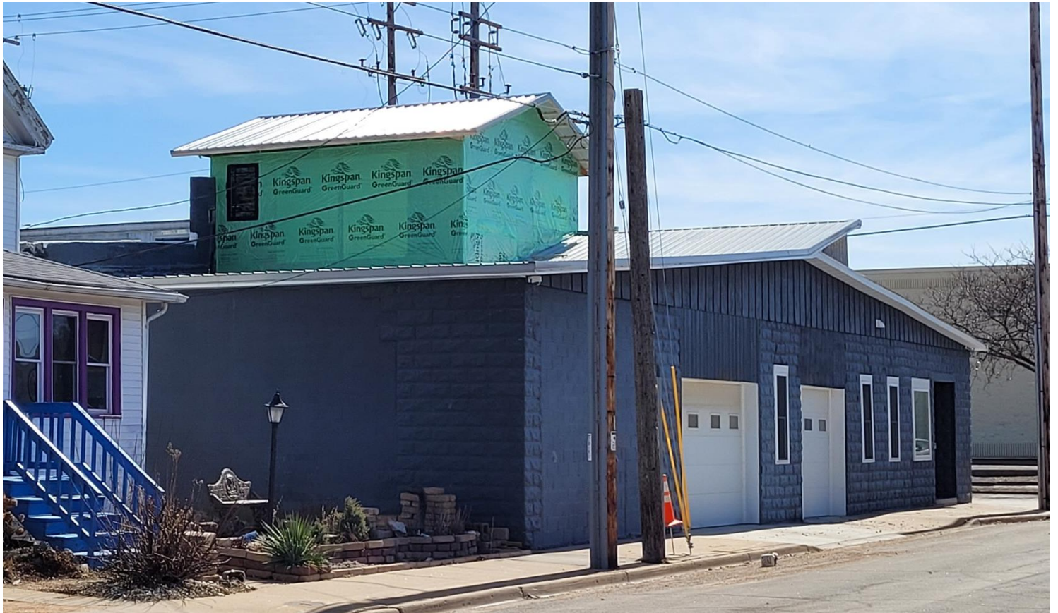
NW Corner of Building – Looking SouthEast
