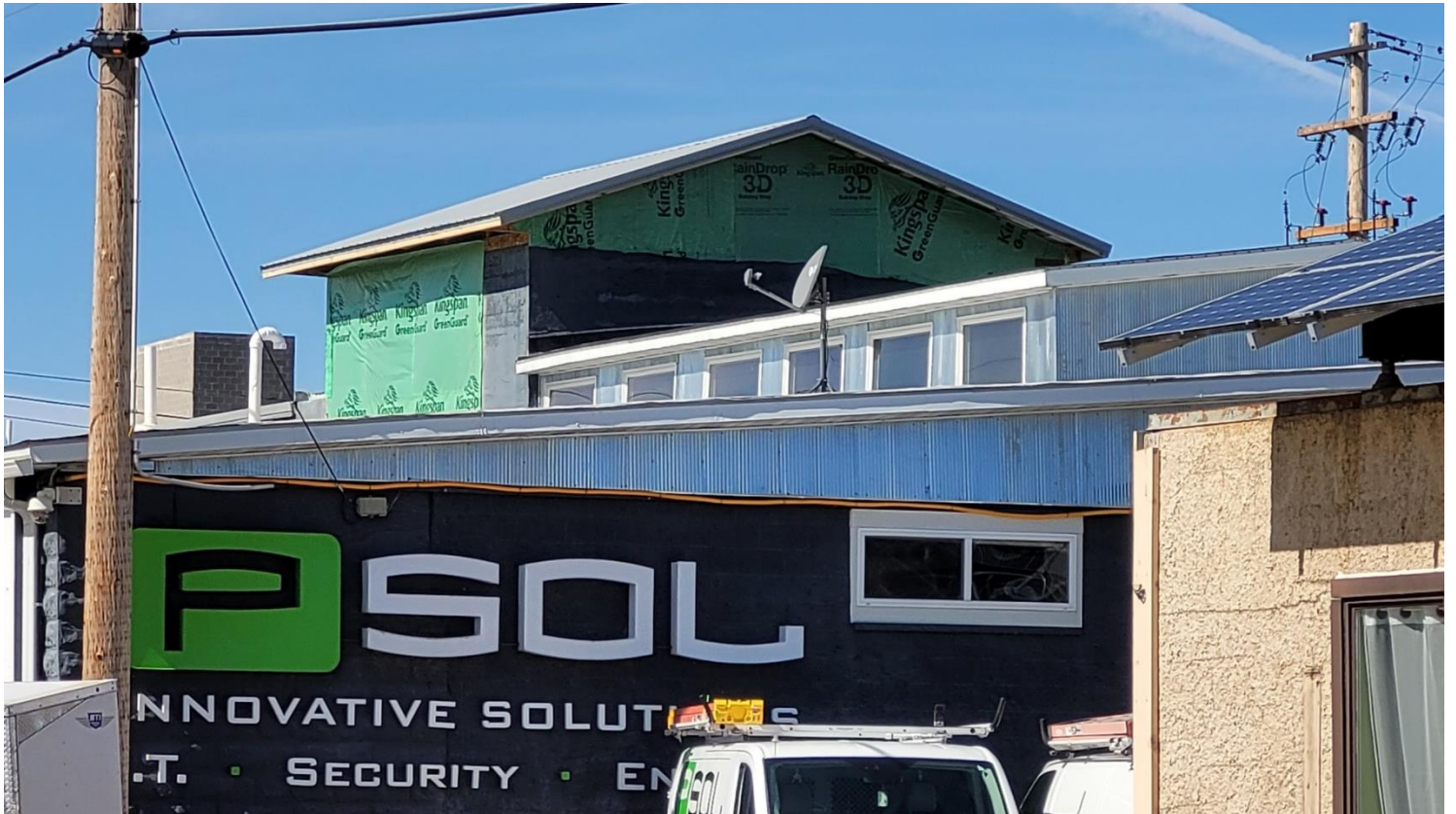
East Wall – Looking West
