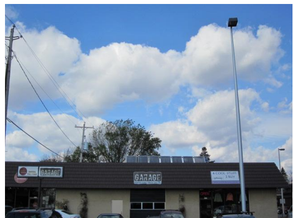
South Side of Building
