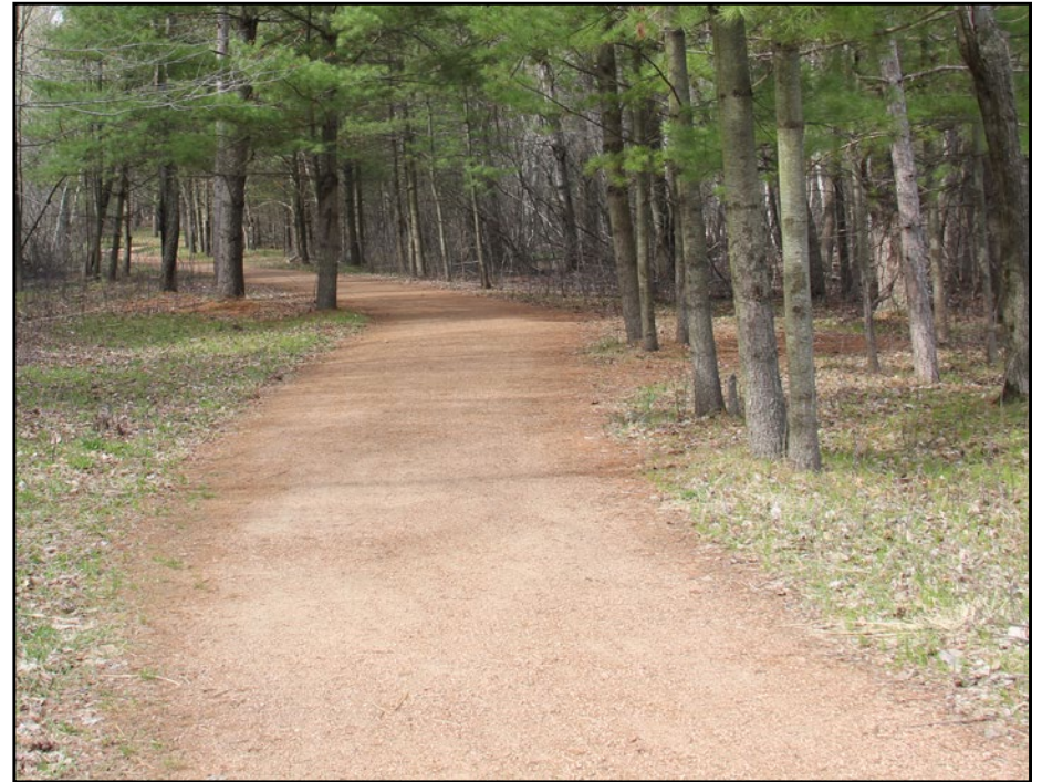
Proposed crushed granite surface
