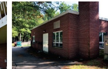
BOILER HOUSE NORTH OF MAIN BUILDING
