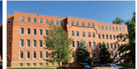
1901 ORIGINAL BUILDING - SOUTH ELEVATION
