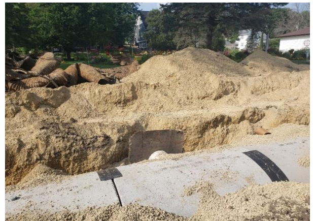
38- by 60-inch HERCP precast fitting for storm inlet; removed existing corrugated pipe in the background.
