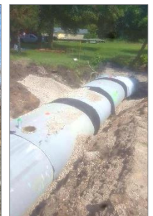
43- by 68-inch HERCP with apron endwall leading to the detention basin.
