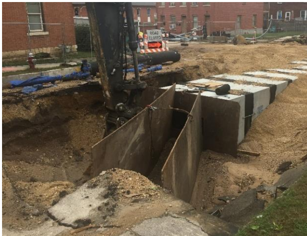
Box culvert construction on 17th Street with temporary stormwater conveyance.
