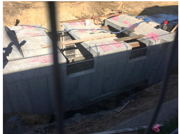
12- by 7-foot box culvert with openings for the permanent high-capacity inlets, full width of the street.
