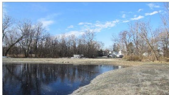
Post construction Ann Street detention basin.
