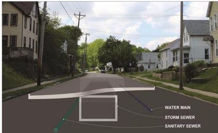
Utility reconstruction on West 17th Street in Dubuque included replacing the existing 54-inch and 60-inch storms sewer system with 10- by 5-foot and 10- by 7-foot concrete box culverts to convey the 25-year storm flow.
