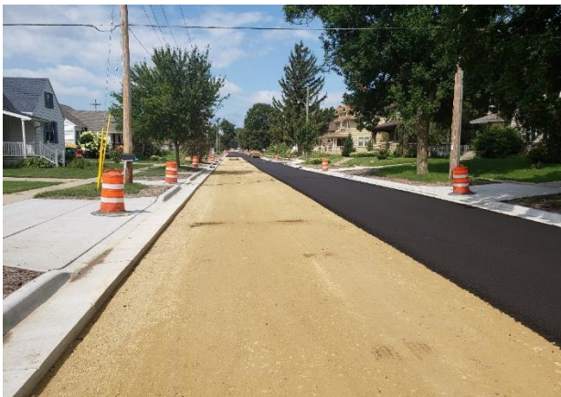
Third Avenue paving looking west (from Third Street).
