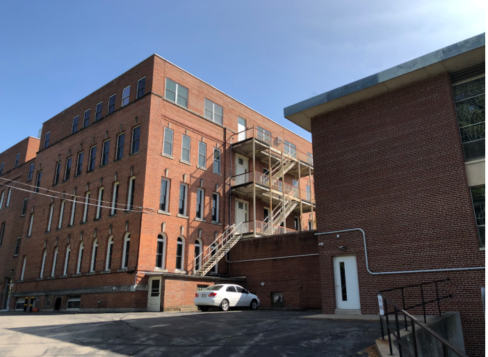
1915 ADDITION & 1964 CHAPEL - NORTH ELEVATION
