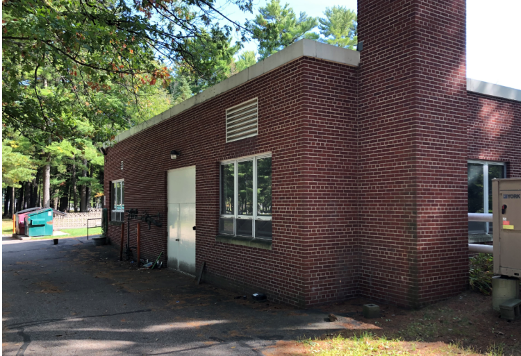
BOILER HOUSE NORTH OF MAIN BUILDING
