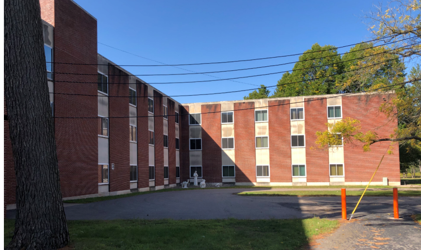
1964 ADDITION - NORTH & EAST ELEVATION
