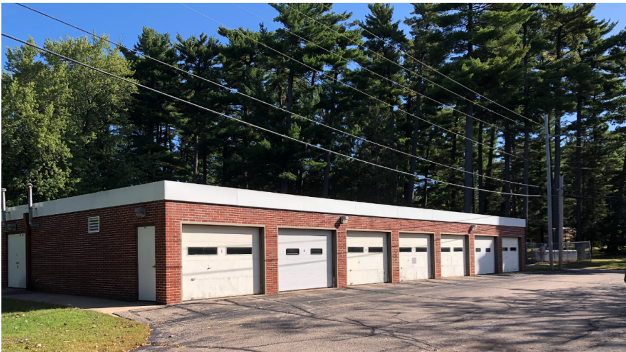
SURFACE GARAGE NORTH OF 1964 BUILDING
