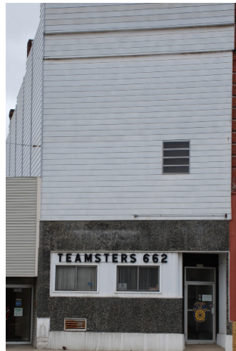
Siding installed over original material
