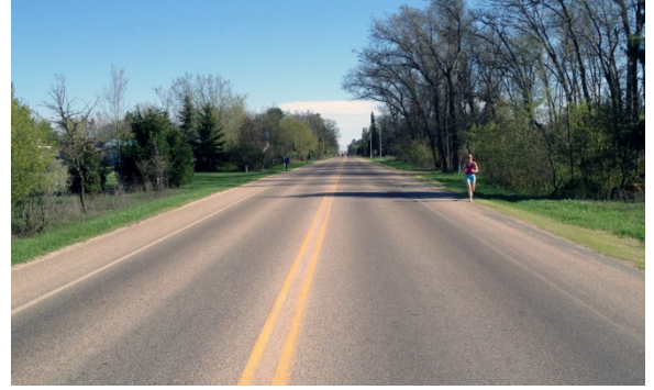
Paved shoulders provide space for pedestrians where sidewalks do not exist.
