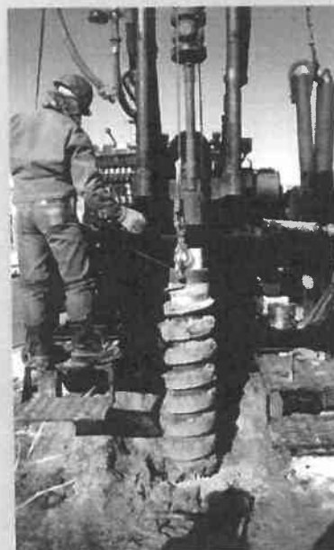
Drilling to monitor for VOCs near a Wisconsin landfill. Photo: DNR
