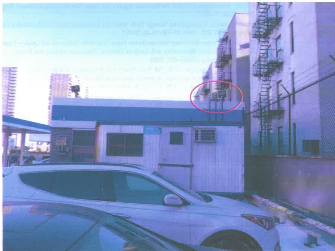
Figure 1: The three vent pipes (enclosed by the red ellipse) on the right side of the convenience store of a gas station are less than 10 m away from the residential building.
