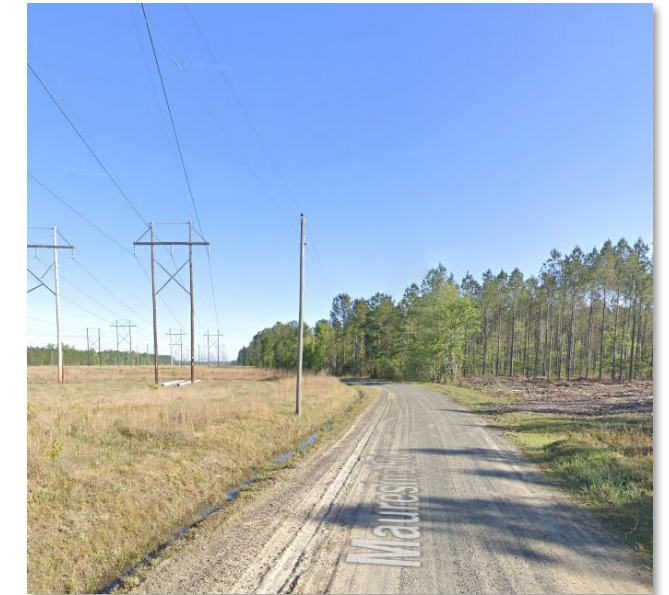
On-site gravel road & transmission ROW
