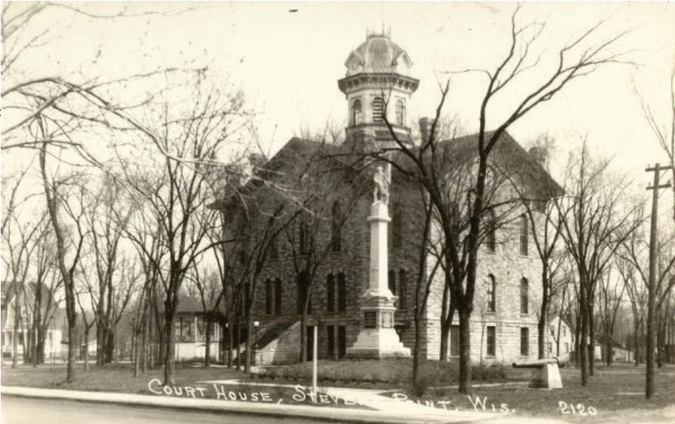
Portage County Courthouse (1910) 94
