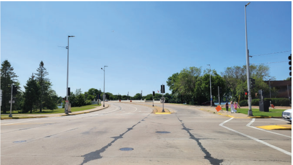
Clark Street, Looking West
