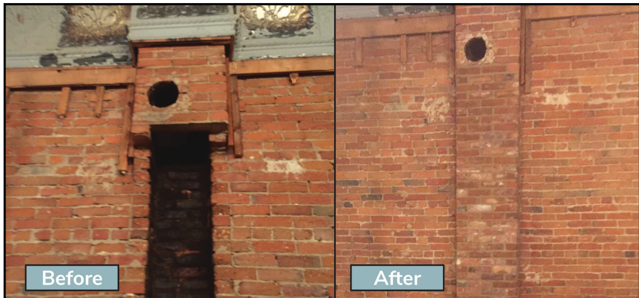
Repairing brickwork to match the existing brickwork.
