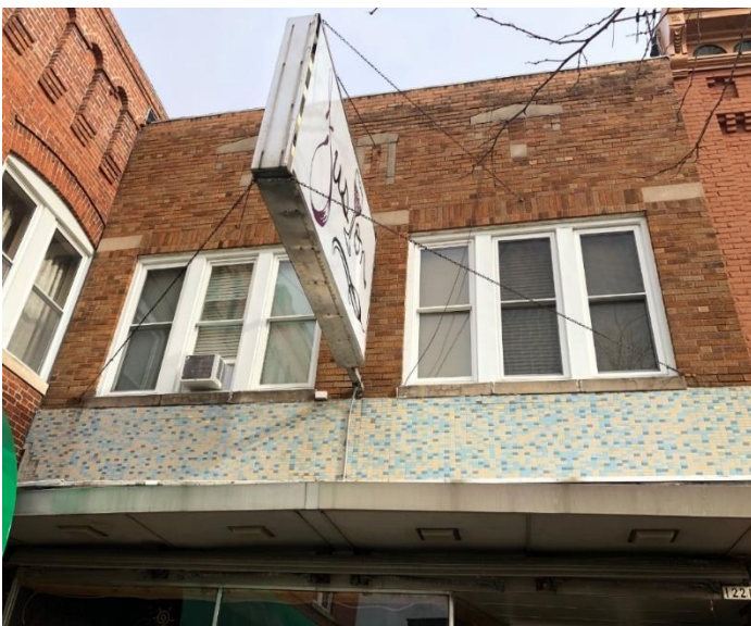
West Façade—Second Floor
