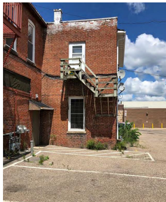
South Façade—Egress Door
