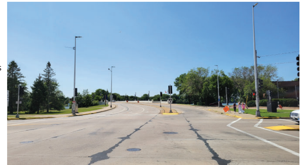
Clark Street, Looking West
