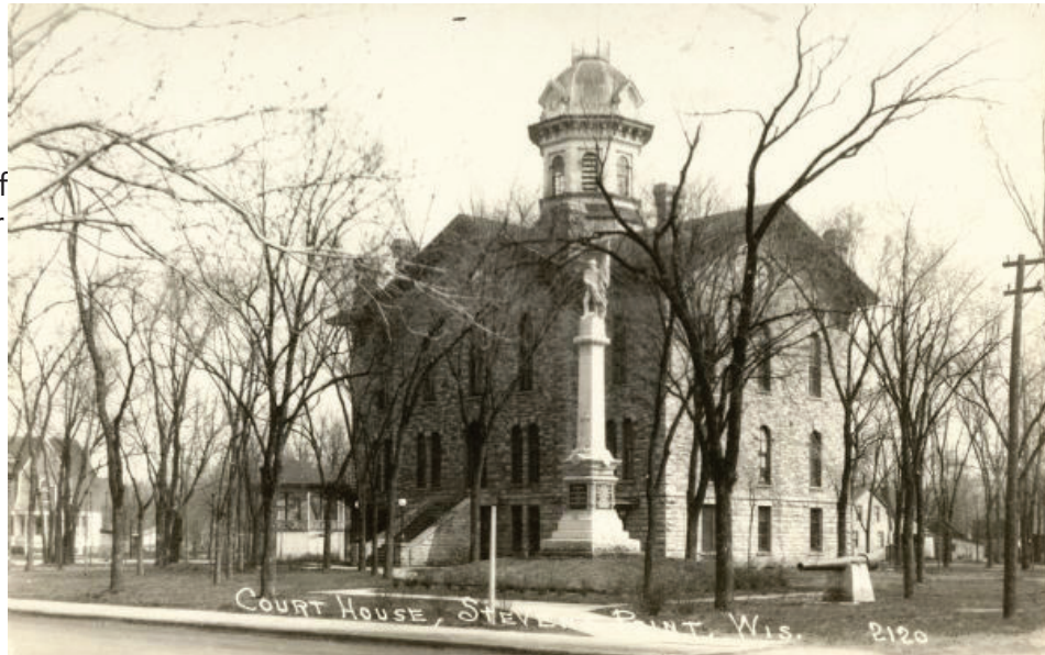
Portage County Courthouse (1910) 94
