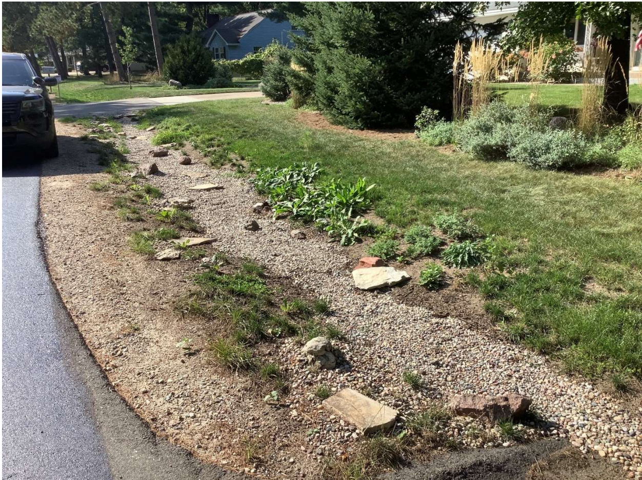
Swale east of driveway, area of non-compliance and the fill material
