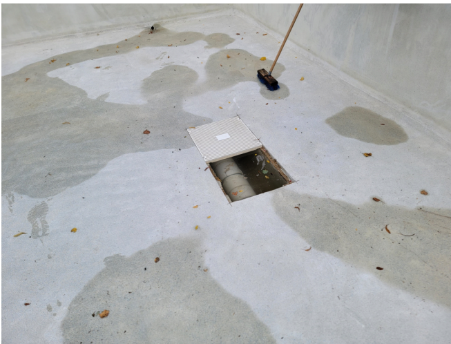
29. VIEW OF MAIN DRAIN IN PLUNGE POOL.
