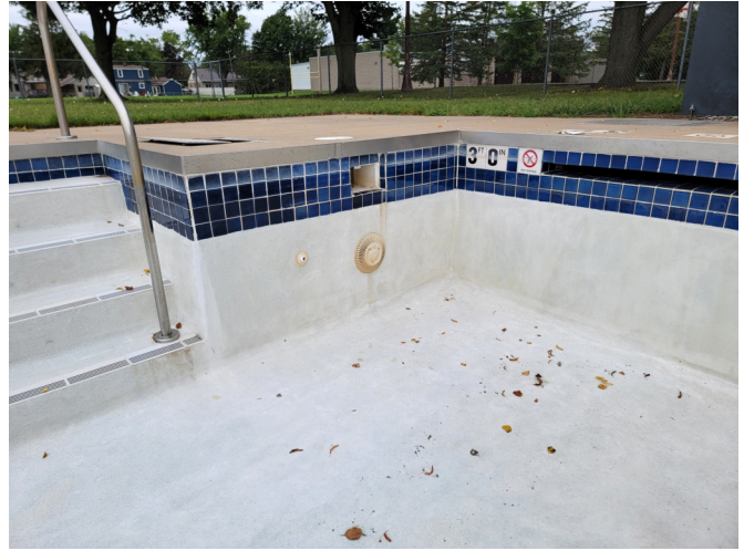
26. VIEW OF SKIMMER AND WEIR OPENING.
