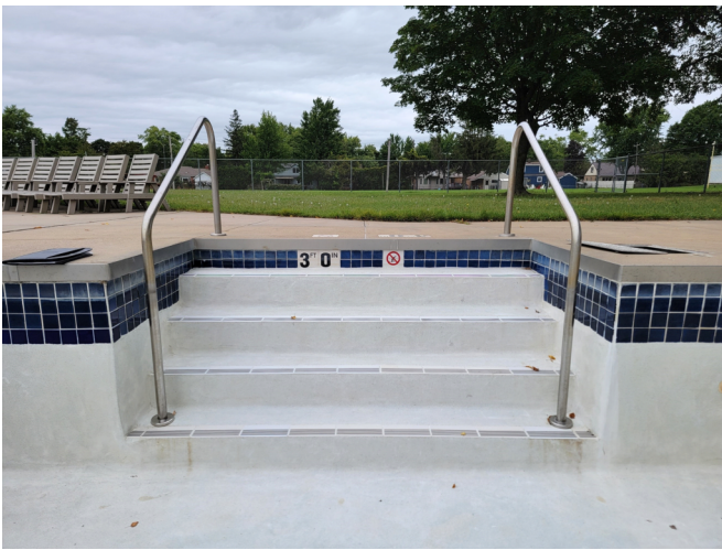
33. VIEW OF PLUNGE POOL STAIRS.
