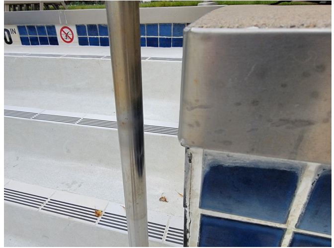
32. VIEW OF STAINLESS STEEL COPING EDGE.
