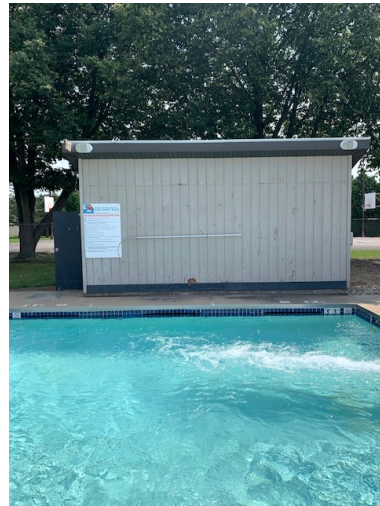
108. VIEW OF SECOND POOL EQUIPMENT BUILDING.
