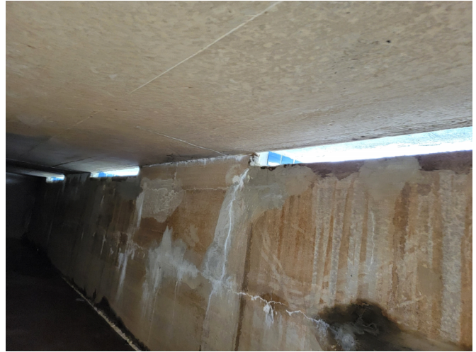
28. VIEW OF INSIDE WEIR TANK.
