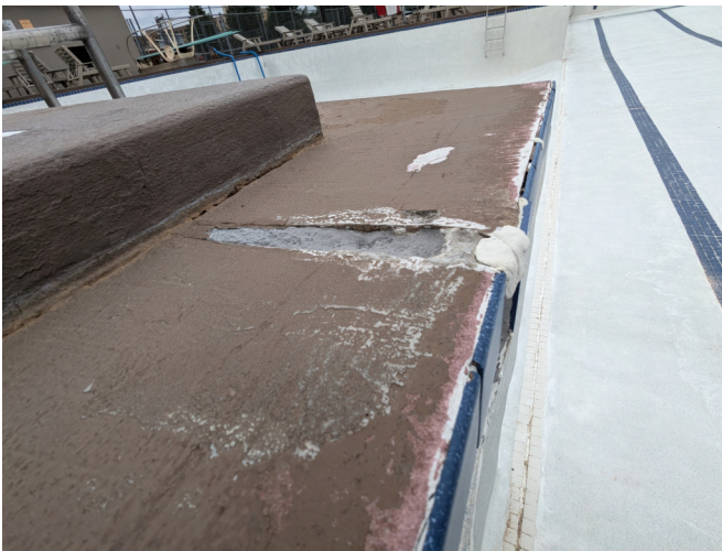
17. VIEW OF EXPANSION JOINT THROUGH GUTTER.
