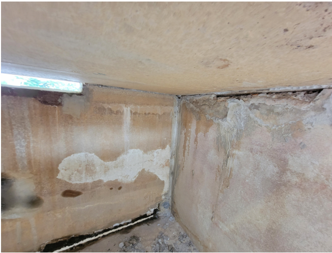
27. VIEW OF INSIDE WEIR TANK.
