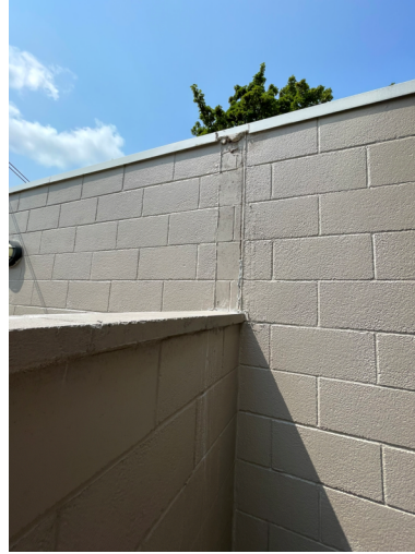
74. VIEW OF ROUGH JOINT AFTER WALL LOWERED.
