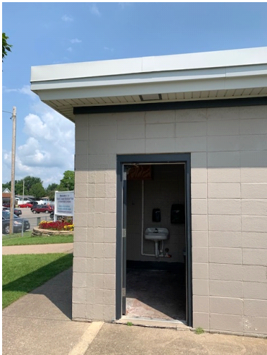
89. VIEW OF PUBLIC RESTROOM.
