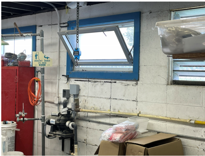
105. VIEW OF WINDOW IN MAIN POOL EQUIPMENT BUILDING.
