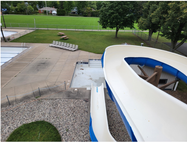
3. VIEW OF PLUNGE POOL FROM SLIDE TOWER.
