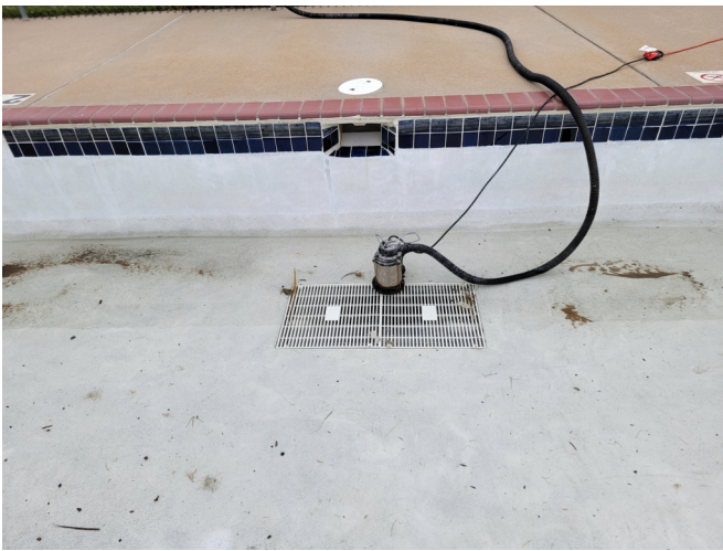
39. VIEW OF WADING POOL MAIN DRAIN.
