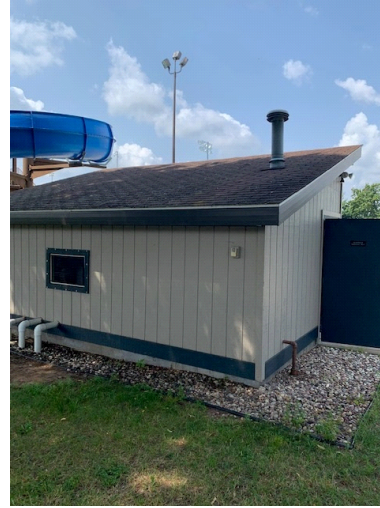
110. VIEW OF BACK OF SECOND EQUIPMENT BUILDING.
