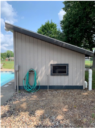
111. VIEW OF SIDE OF SECOND EQUIPMENT BUILDING.
