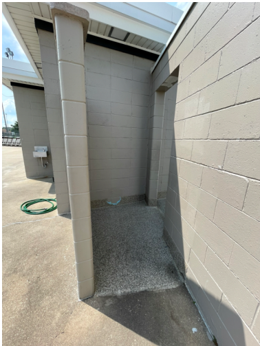
71. VIEW OF LOCKER ROOM WALKWAY TO POOL AREA.
