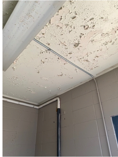
94. VIEW OF CEILING IN PUBLIC RESTROOM.
