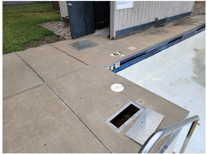
8. VIEW OF NARROW DECK BY PLUNGE POOL.
