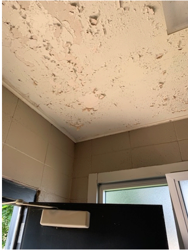
93. VIEW OF CEILING IN PUBLIC RESTROOM.
