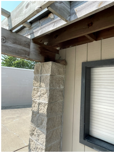
99. VIEW OF SNACK BUILDING COLUMN
