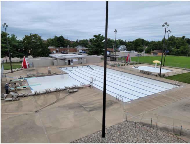
55. VIEW OF LIGHT POLE.
