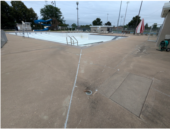
13. VIEW OF MAIN POOL FROM NW CORNER.
