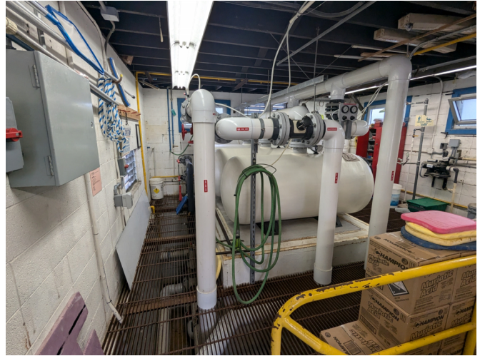
46. CORROSION ON STAIRS AND GRATING
