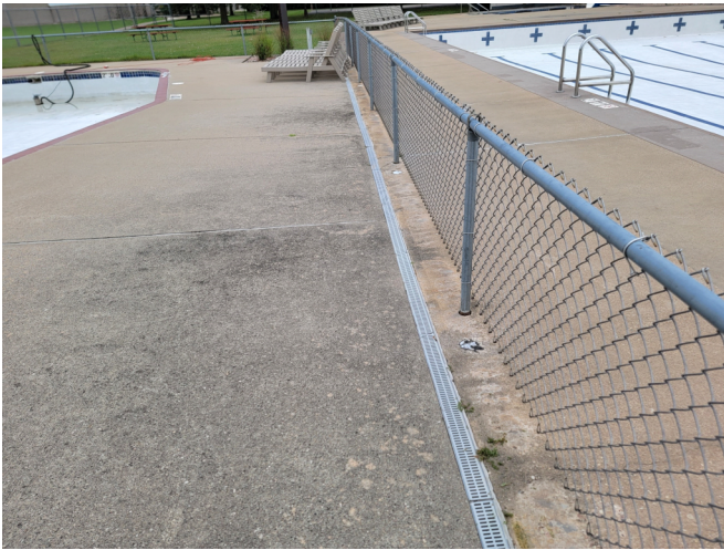
9. VIEW OF DECK DRAIN BETWEEN MAIN AND WADING POOLS.
