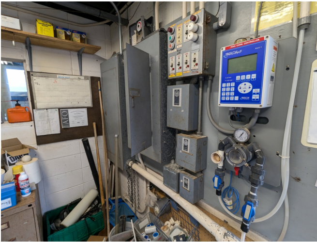
45. VIEW MAIN POOL CHEMICAL CONTROLLER.
