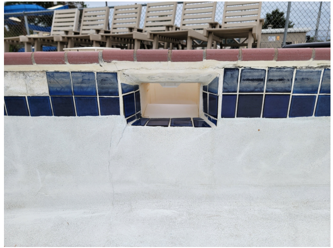
38. VIEW OF SKIMMER IN WADING POOL.
