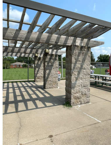
96. VIEW OF PERGULA AT SNACK BUILDING.
