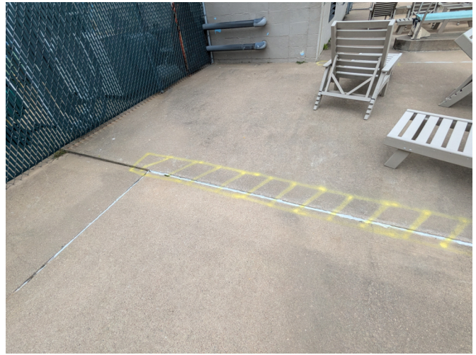
44. VIEW OF POOL DECK WITH EXPOSED HEATER PIPING.
