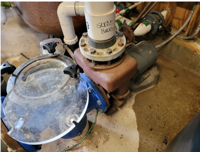
47. VIEW OF PLUNGE POOL RECIRCULATION PUMP.
