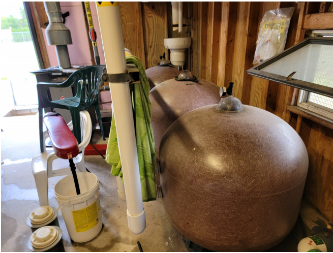
49. VIEW OF PLUNGE POOL FILTERS.
