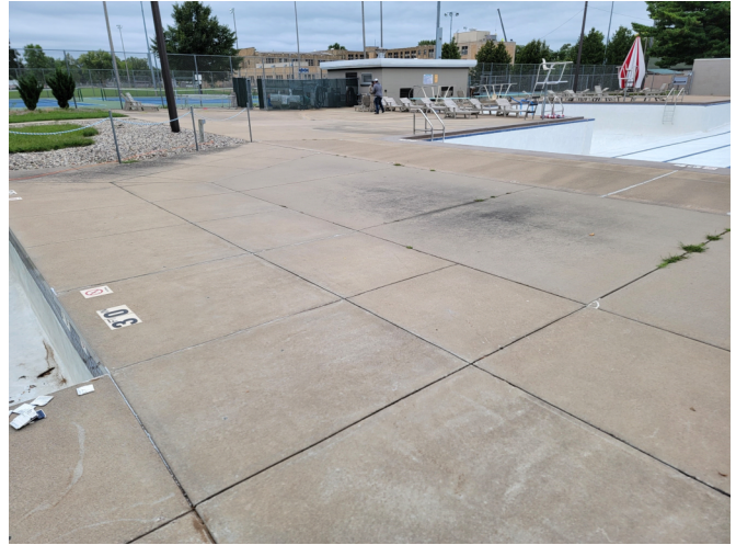
10. VIEW OF DECK BETWEEN MAIN AND PLUNGE POOLS.
