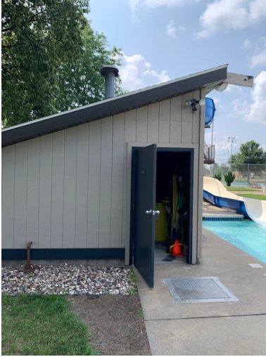
109. VIEW OF DOOR TO SECOND EQUIPMENT BUILDING.
