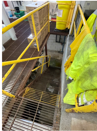
106. VIEW OF STAIRS IN MAIN POOL EQUIPMENT BUILDING.
