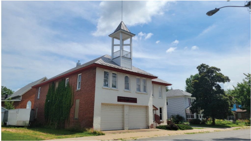
Historic Fire House #2
