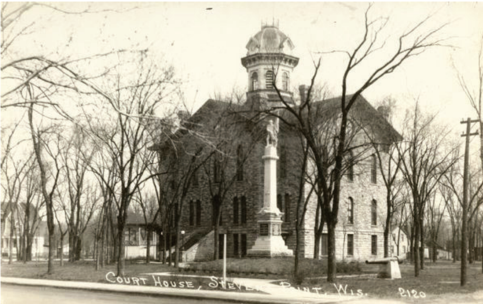
Portage County Courthouse (1910) 94
