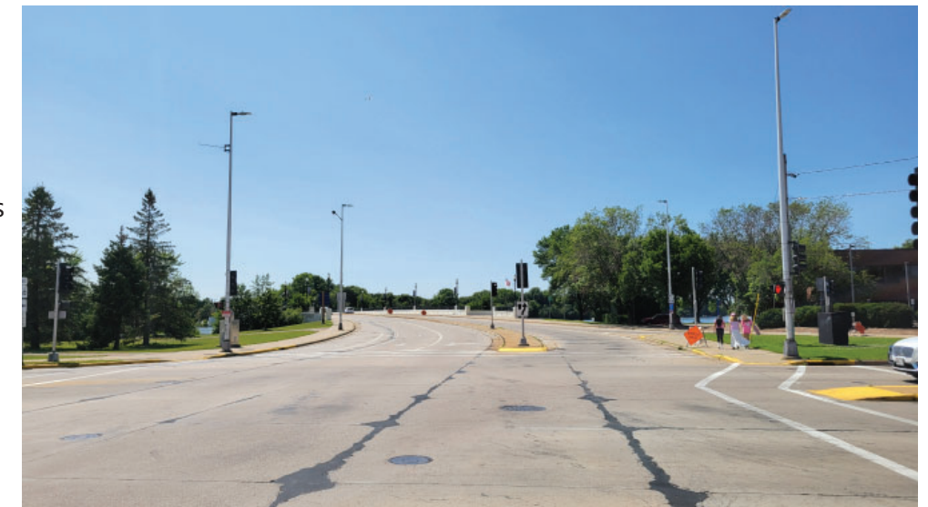
Clark Street, Looking West
