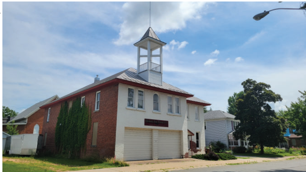
Historic Fire House #2
