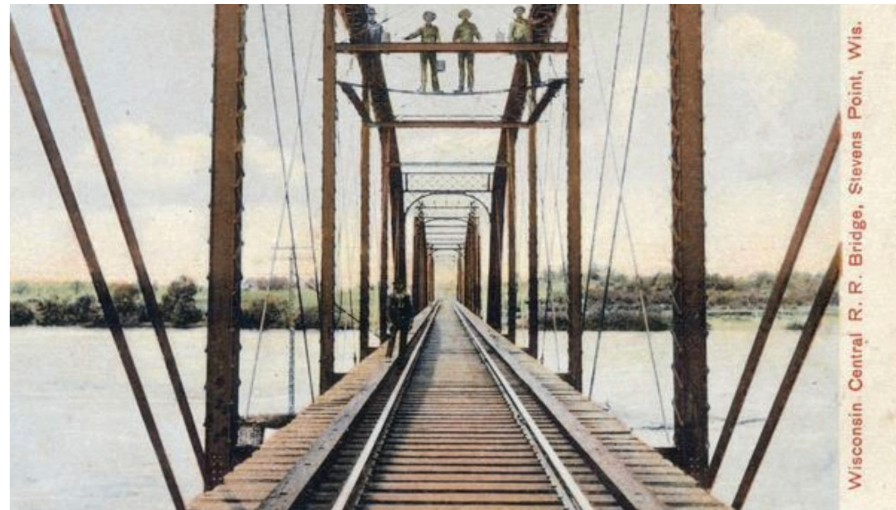
Canadian National Railroad Bridge Over the Wisconsin River 18
