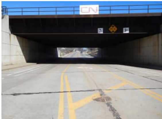
Narrowing the street width of Michigan Avenue will be considered during design.
