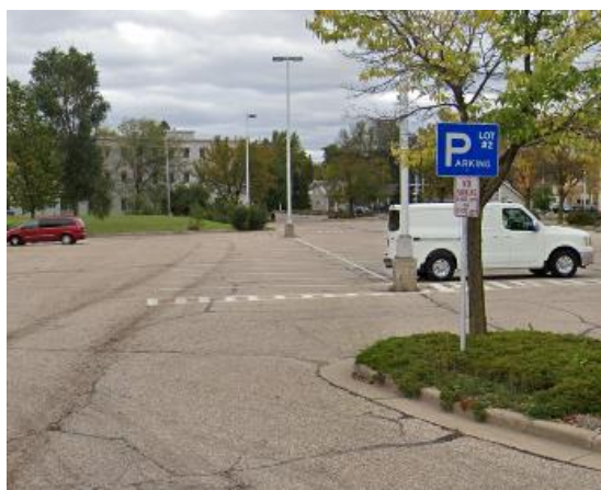
Inadequate signage and wayfinding.
