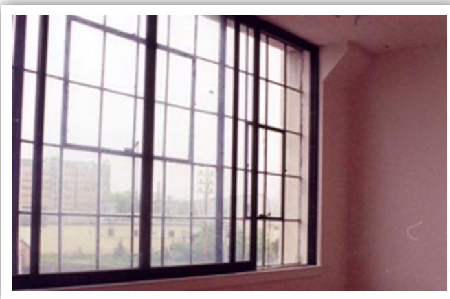
Recommended Original metal windows were retained and made operable during the rehabilitation of this historic mill complex. Installing patio slider doors as interior storm windows was a creative and successful solution to improve the energy efficiency of the existing windows.
