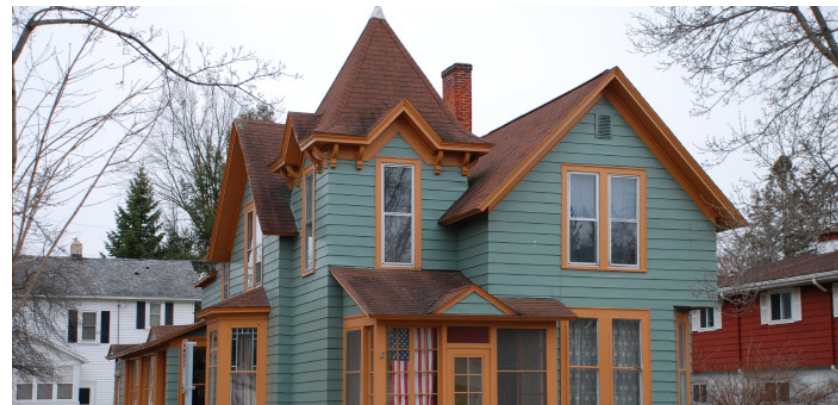
Steeply pitched gable roof
