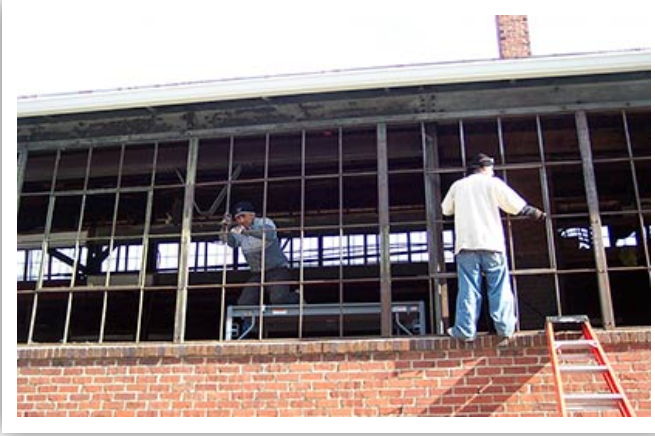
Recommended Original metal windows were appropriately repaired as part of the rehabilitation of this historic industrial building. During rehabilitation.
