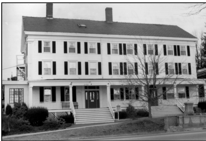
Tavern after rehabilitation before appropriate entrance installed.
