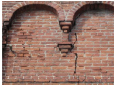
Deteriorated masonry
