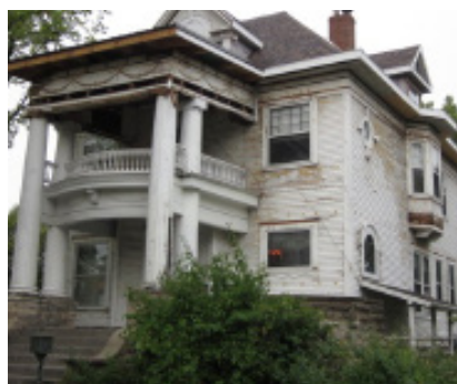
Siding removed revealing original woodwork.
