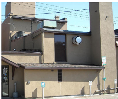
A stucco-like material (EIFS) installed over brick.
