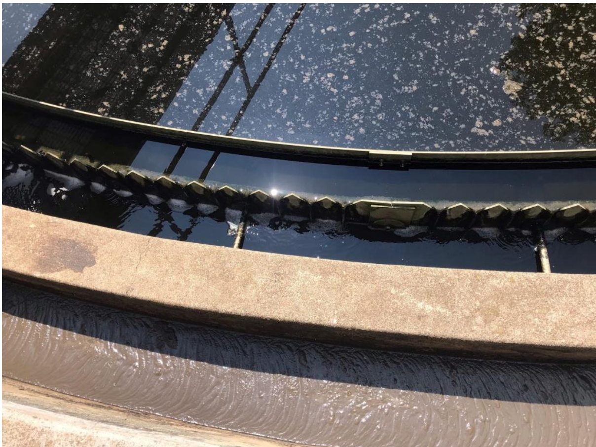
Photo 26: North Clarifier Weir
