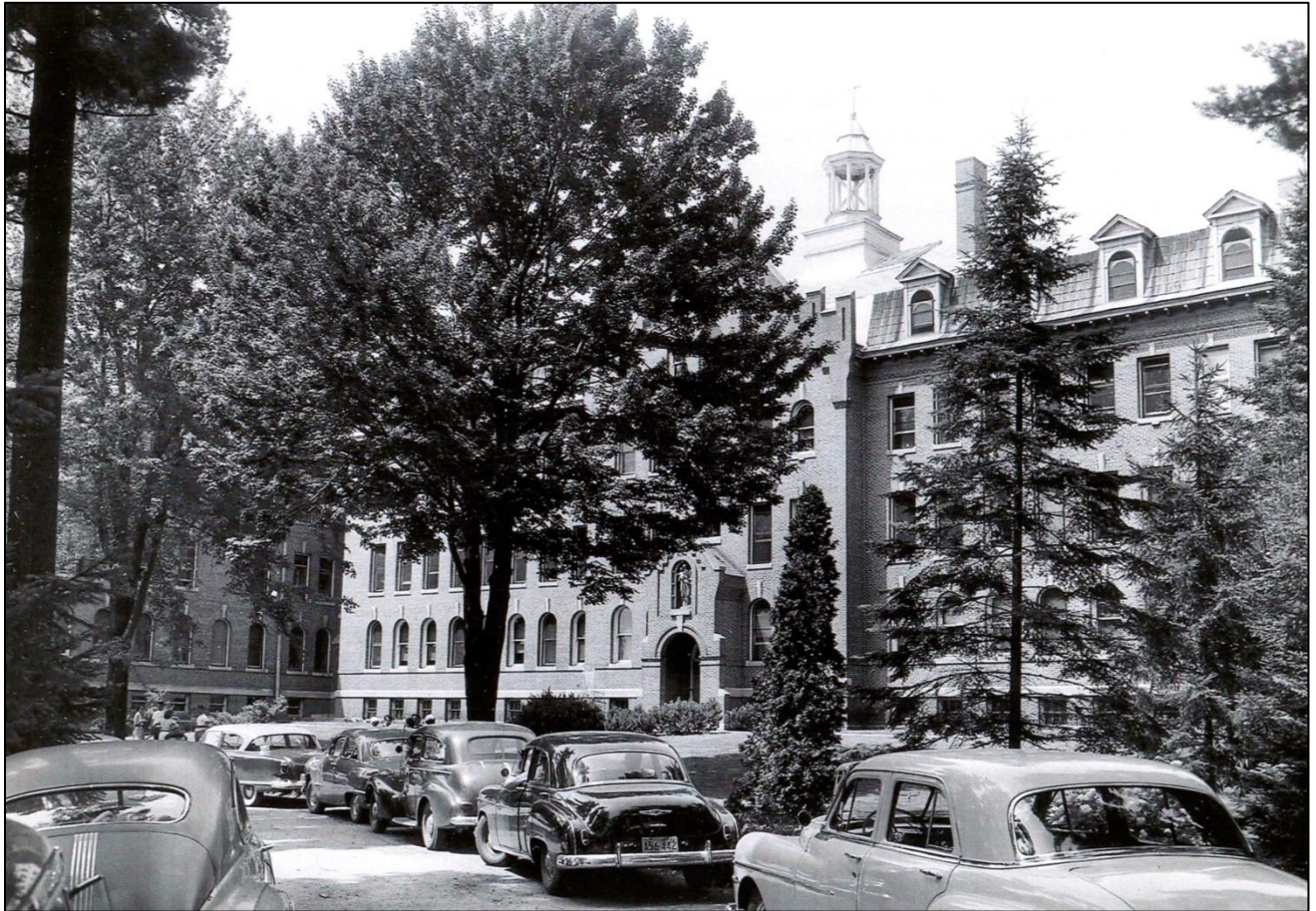
Figure 5: 1903 convent with 1916 addition on left, undated photograph (image retained by the Sisters of St. Joseph of the Third Order of St. Francis)
