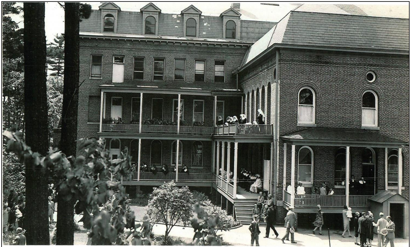
Figure 4: Rear elevation of 1903 convent showing original chapel wing on right, undated photograph (image retained by the Sisters of St. Joseph of the Third Order of St. Francis)
