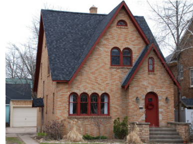
Residential window and doors
