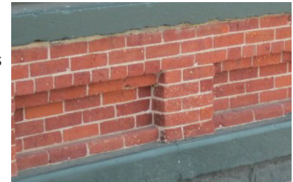
Re-pointed and painted masonry
