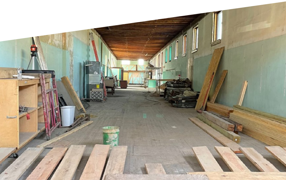
Renovation in progress in Marshalltown Central Business District — Marshalltown, Iowa.
