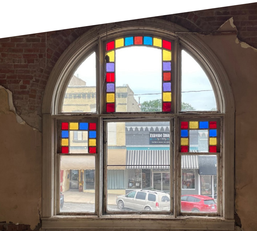
Efforts in Corning, Iowa are underway to renovate the historic Widener building (built 1896) to add ground-floor commercial and upper-floor residential units. Main Street Corning, Iowa
