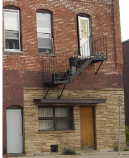
Fire escape and access accommodations should be placed on rear elevations if possible.
