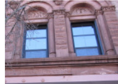
Second floor commercial windows
