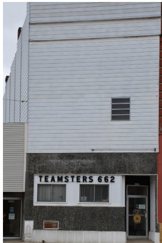
Siding installed over original material
