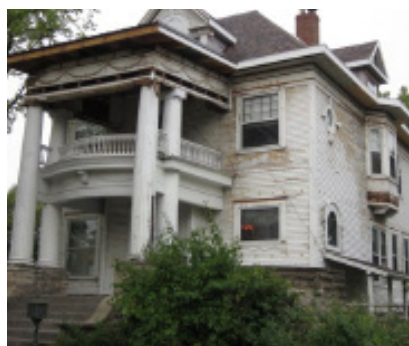
Siding removed revealing original woodwork.
