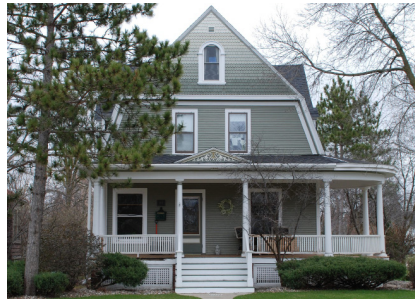
Existing decks should be maintained appropriately.
