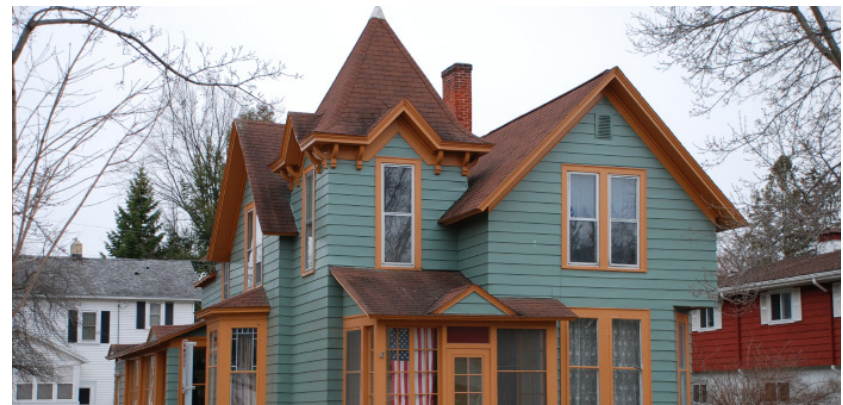
Steeply pitched gable roof
