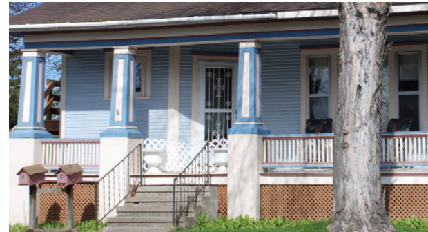
Well maintained porches preserve significant architectural features
