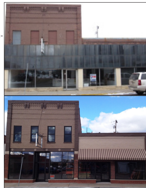
Reconstructed storefront based on original design
