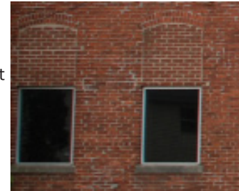
Covering or filling in original window or door openings is not recommended
