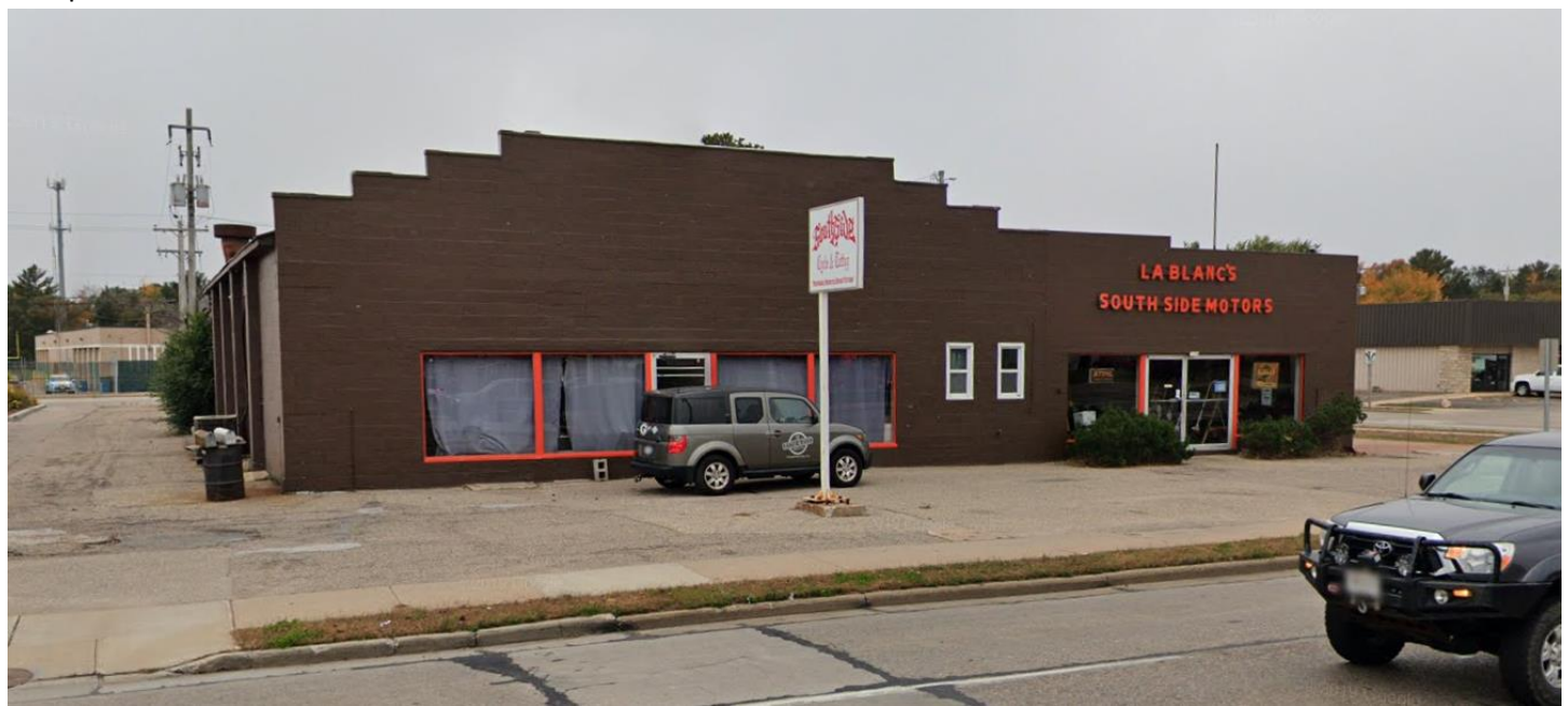
The applicant conducting business operations at 3310 Church Street (circa October 2019).
