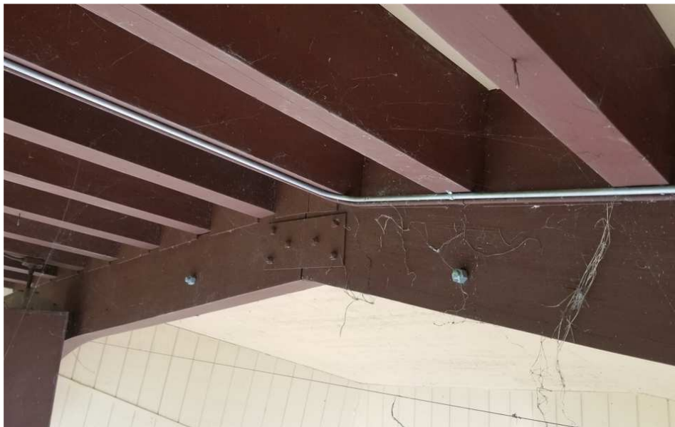
Figure 23 - Typical Rafter End Bearing at Front Face of Secondary Arch
