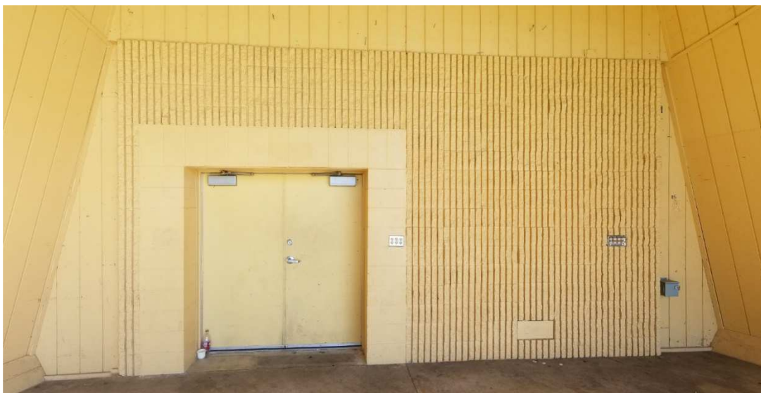
Figure 5 – Fluted Masonry Wall at Back of Stage
