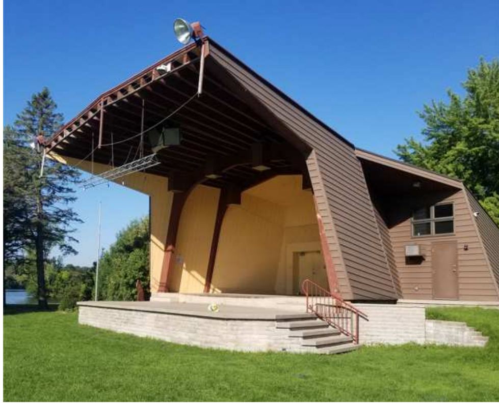
Figure 3 - View from East, Looking West
