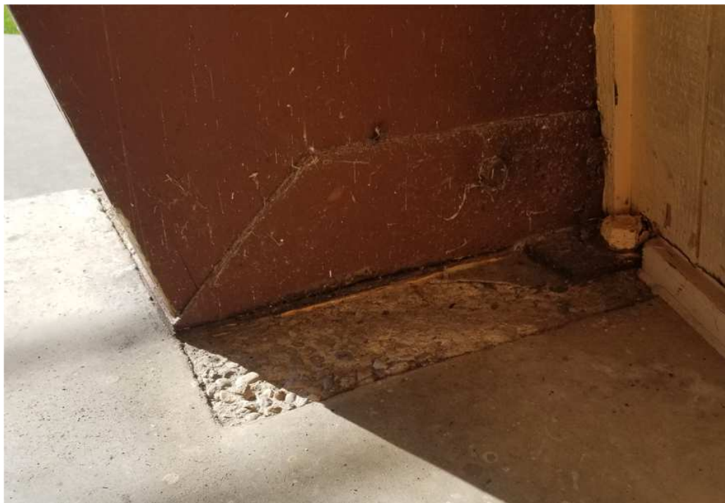
Figure 15 - Good Finish Condition at Back Face of Southwest Arch Base
