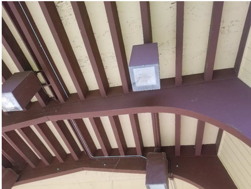
Figure 26 – Typical Underside of Roof Deck over Stage
