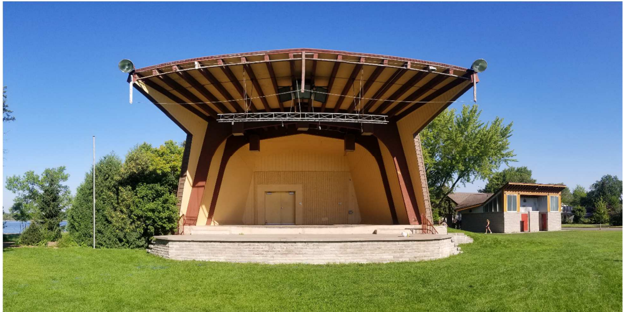
Figure 1 - View of Bandshell from Southeast
