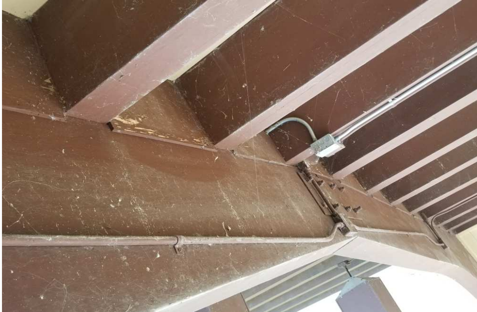
Figure 24 - Typical Rafter Bearing Over Primary Arch
