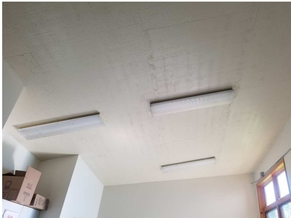
Figure 29 - Plywood Sheathed Ceiling in Addition - No Staining Noted
