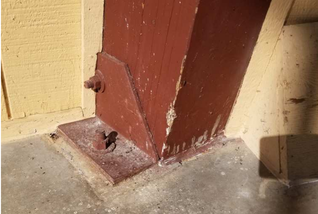
Figure 17 - Southwest Base of Secondary Arch
