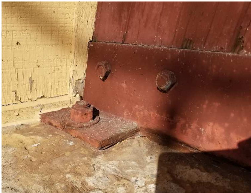
Figure 9 - Front Side of Southwest Anchorage for Primary Arch
