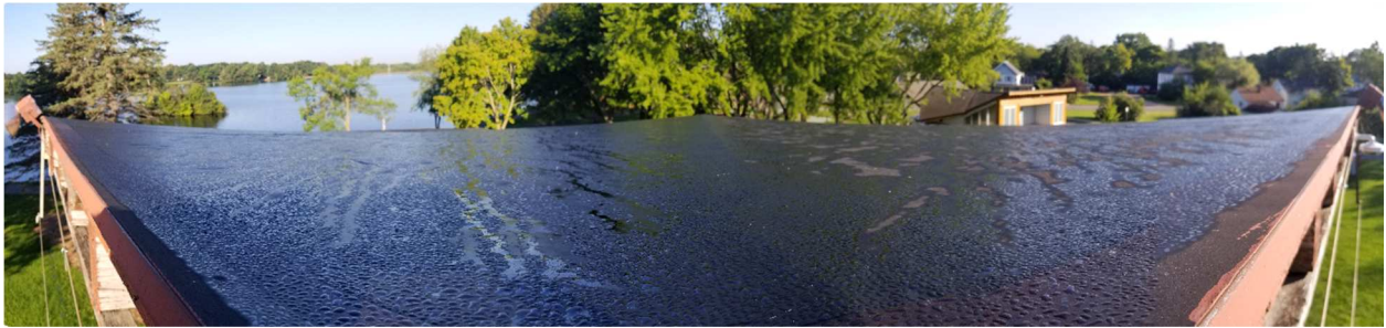
Figure 25 – Panoramic of Roof Over Stage Area
