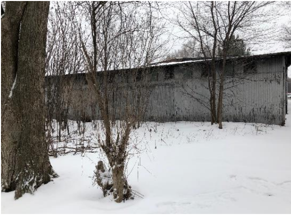
Structure Three: Storage Warehouse
