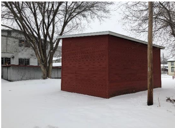
Structure Five: Storage Shed
