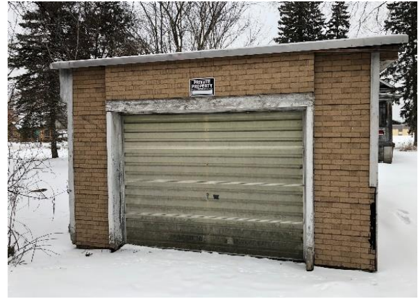
Structure Four: Residential Garage
