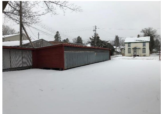
Structure Six: Storage Shed
