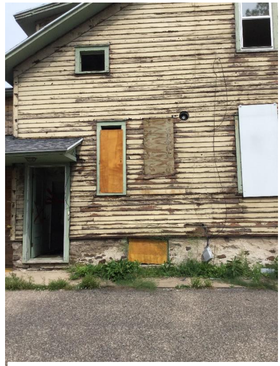
Temporary Coverings Over Window Openings
