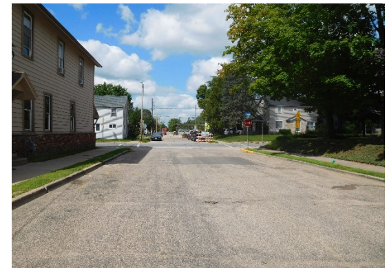
Maintaining accessibility to business and limiting construction impacts are crucial.
