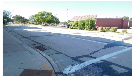
Traffic control and detouring will be critical at Portage Street and Second Street.
