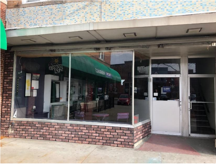
West Façade—First Floor
