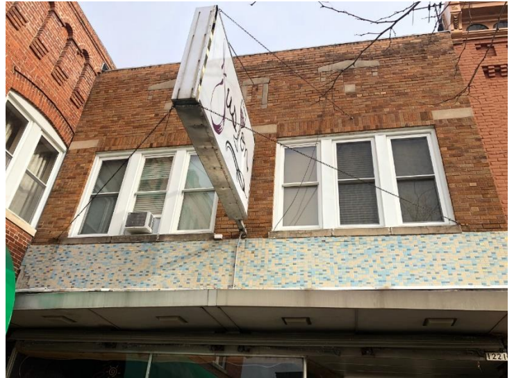
West Façade—Second Floor
