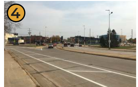
CLARK ST. BRIDGE, LOOKING EAST
