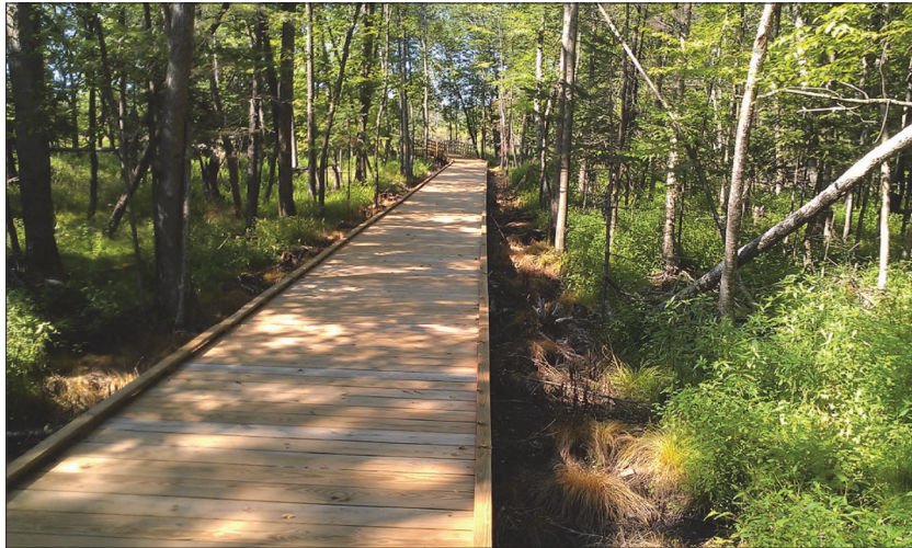
<12" ABOVE GRADE - BOARDWALK W/ RUB RAIL
