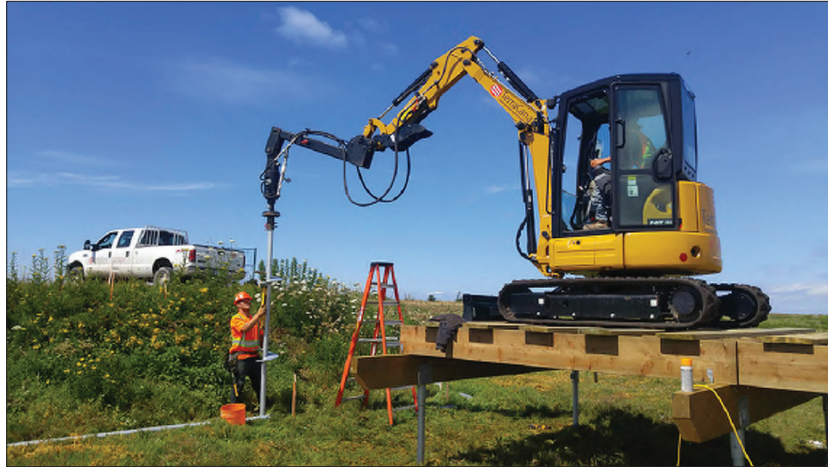
HELICAL PILE FOUNDATION - RECOMMENDED
