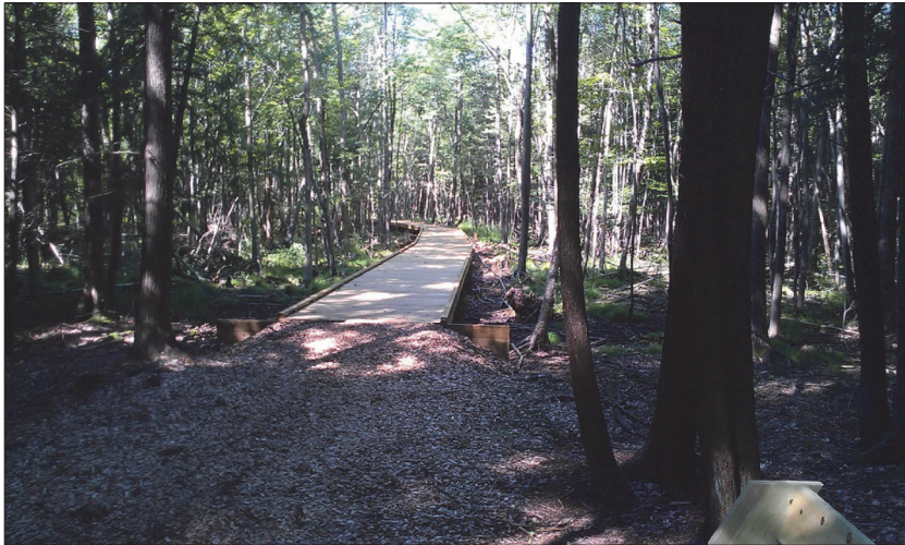
<12" ABOVE GRADE - BOARDWALK W/ RUB RAIL
