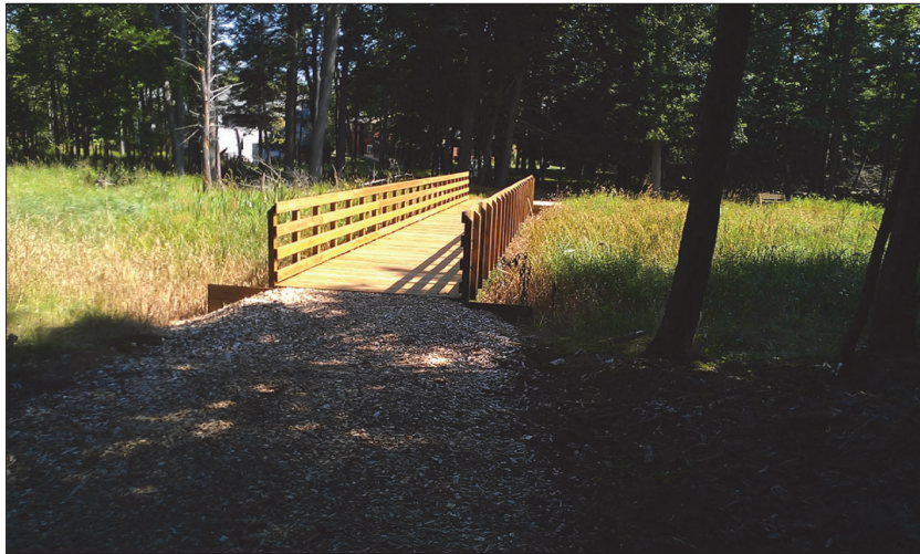
>12" ABOVE GRADE - BOARDWALK W/ RAILING
