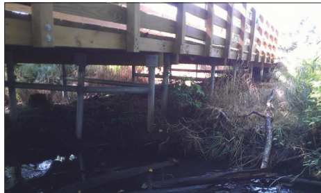
PIPE PILE FOUNDATION
