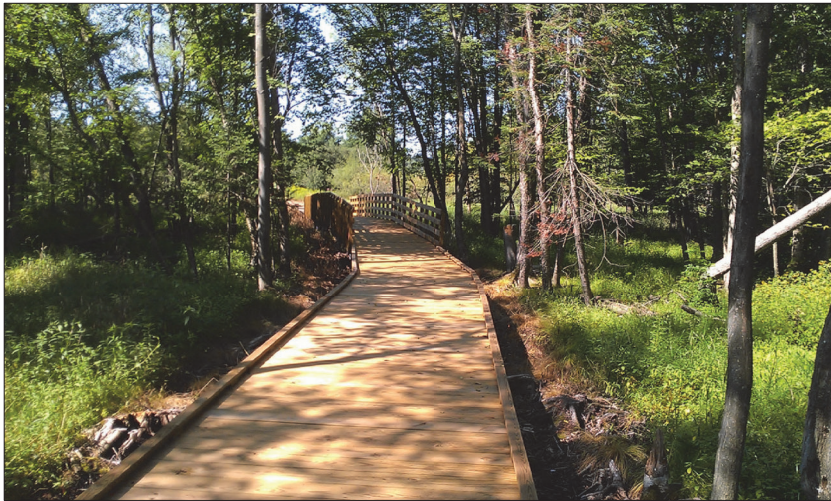
BOARDWALK W/ RUB RAIL TRANSITIONING TO RAILING
