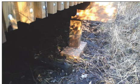
SPREAD FOOTING FOUNDATION
