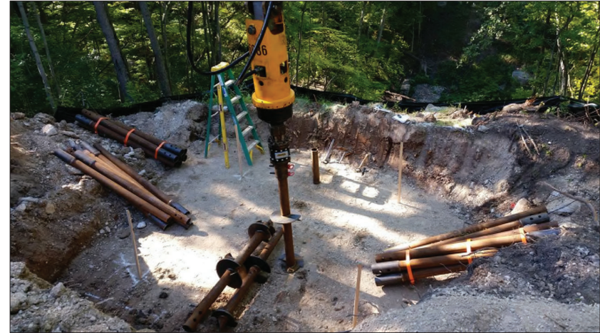
HELICAL PILE FOUNDATION - RECOMMENDED
