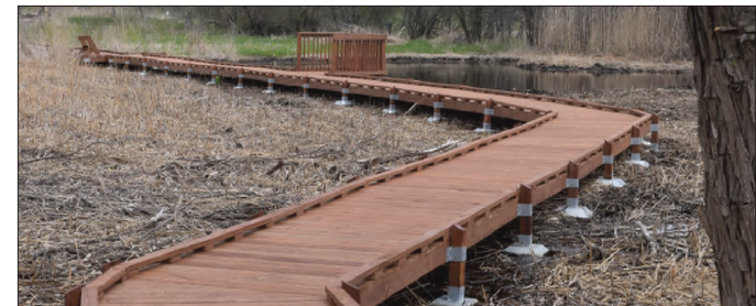
METAL PAN PILE FOUNDATION
