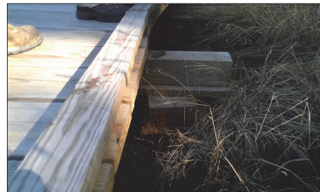
SPREAD FOOTING FOUNDATION
