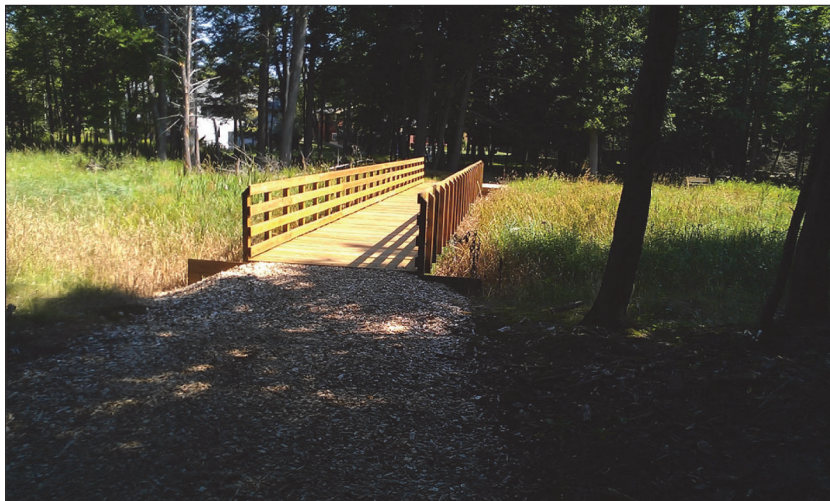
>12" ABOVE GRADE - BOARDWALK W/ RAILING
