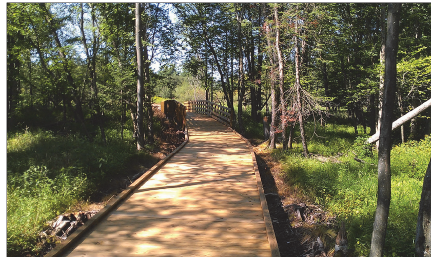
BOARDWALK W/ RUB RAIL TRANSITIONING TO RAILING
