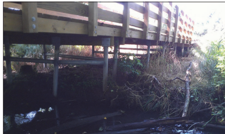
PIPE PILE FOUNDATION
