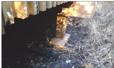
SPREAD FOOTING FOUNDATION
