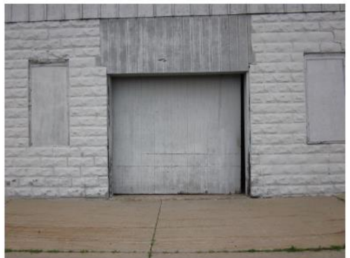
2014 - West Façade Garage Before
