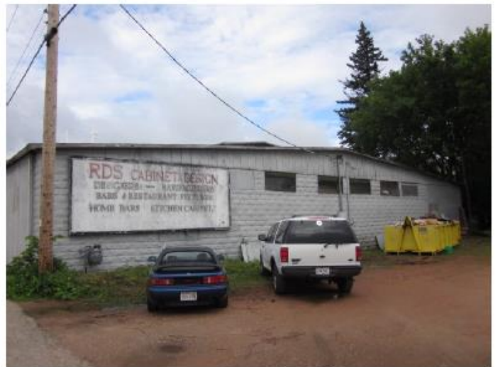
2014 - East Façade Before
