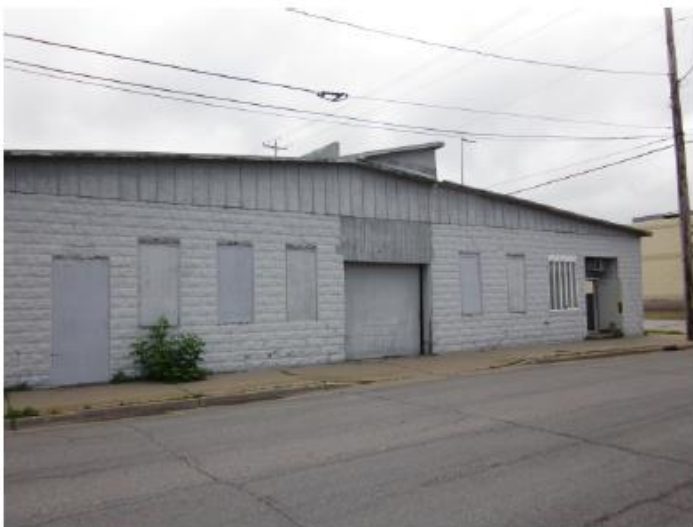
2014 - West Façade Before
